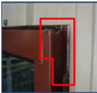
Figure 6.1 Head to Jamb junction
