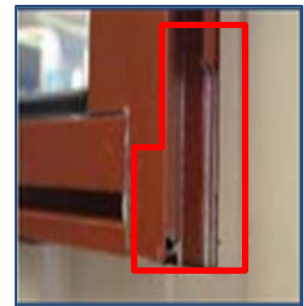
Figure 6.2 Sill to jamb junction
